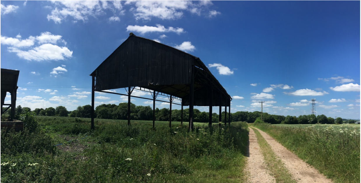
Photo 2: View of East (end) elevation of Barn No. 2
