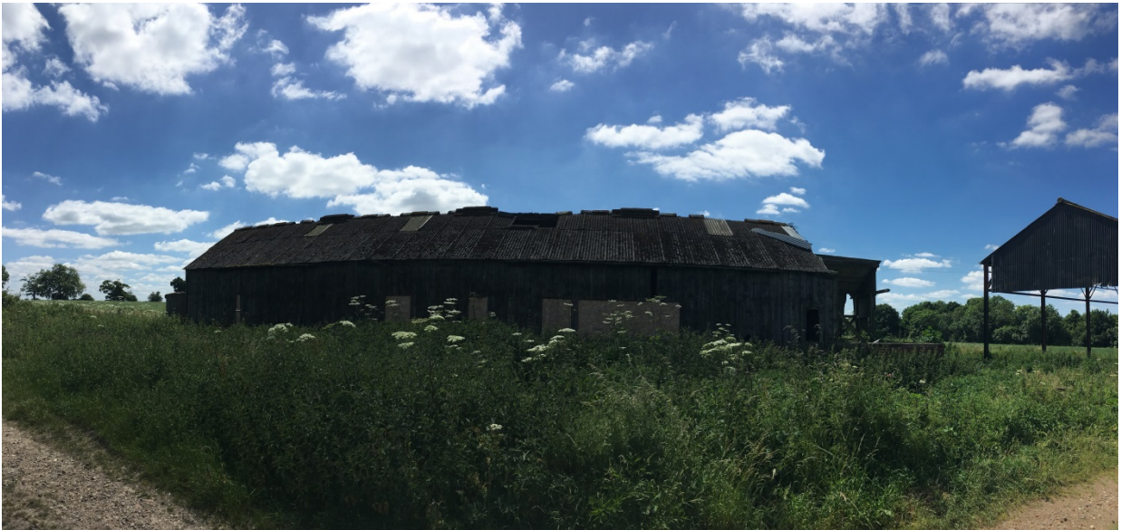
Photo 6: View of South (side) elevation of Barn No. 1
