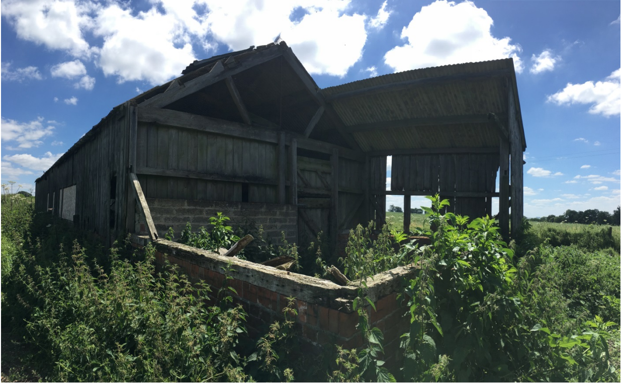
Photo 7: View of West (end) elevation of Barn No. 1
