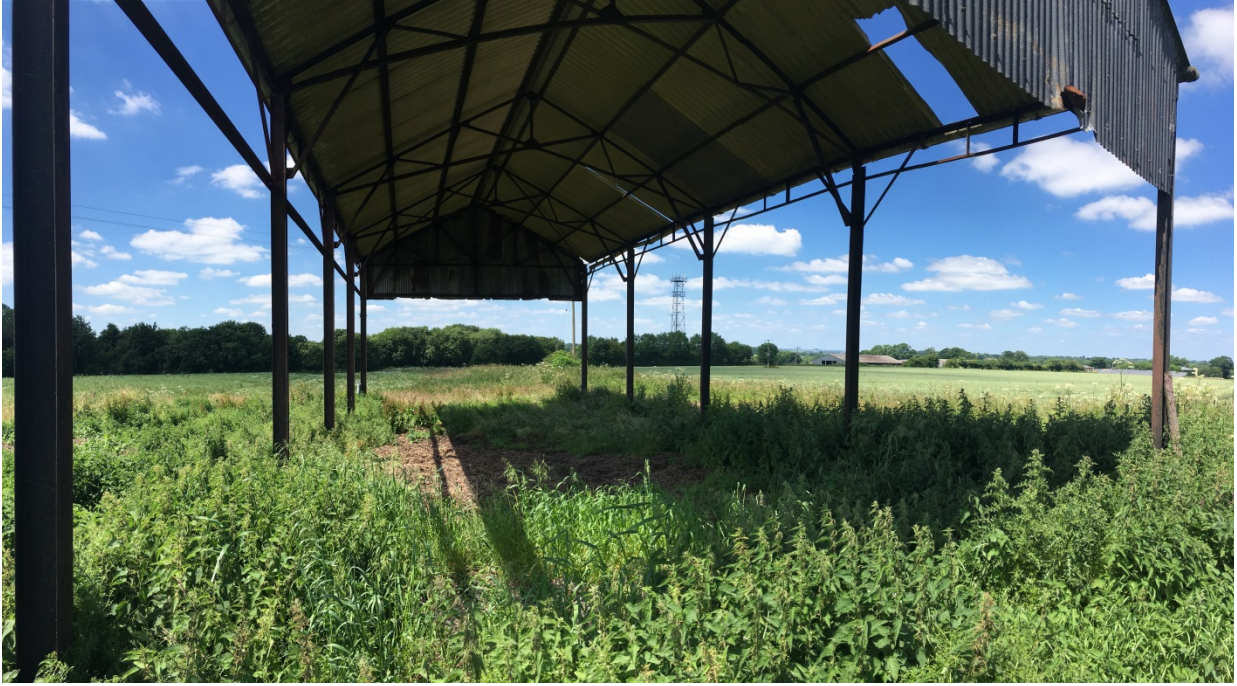
Photo 3: View inside Barn No. 2
